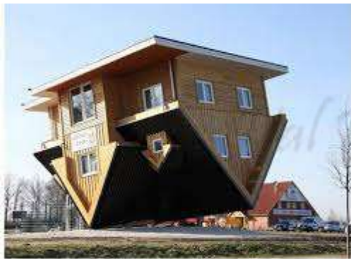
This upside-down building known as "Crazy House" was built in Ellwangen, Germany, as a tourist attraction. www.dailymail.com
